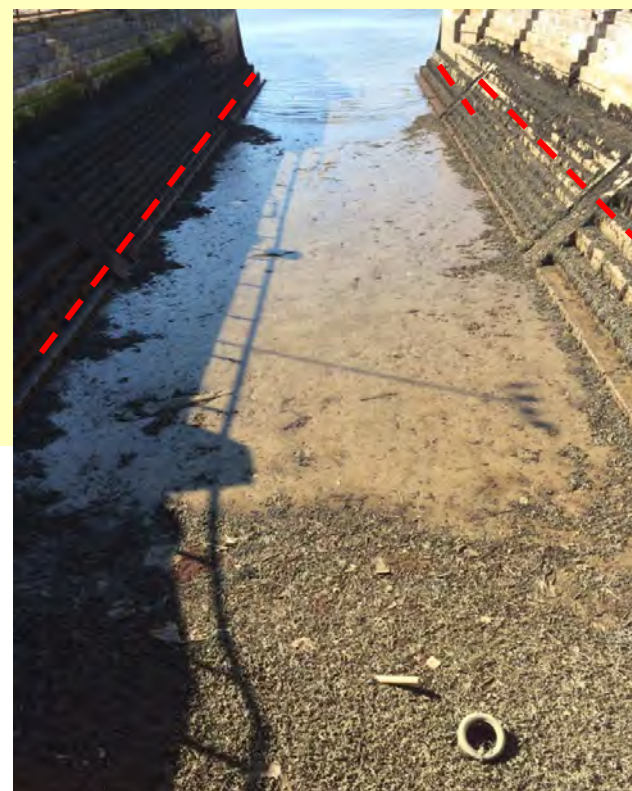
Photo of Dock 4 during low spring tide showing silt level Source: PCC
